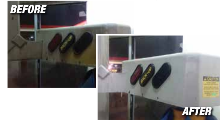
Soap Scum on Painted Metal at Car Wash
