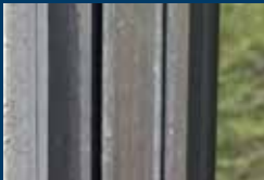
Before cleaning bronze anodized aluminum window frames
